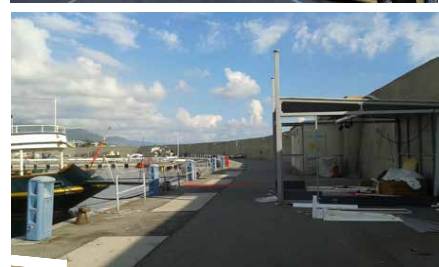
D | Sea Barrier wall
