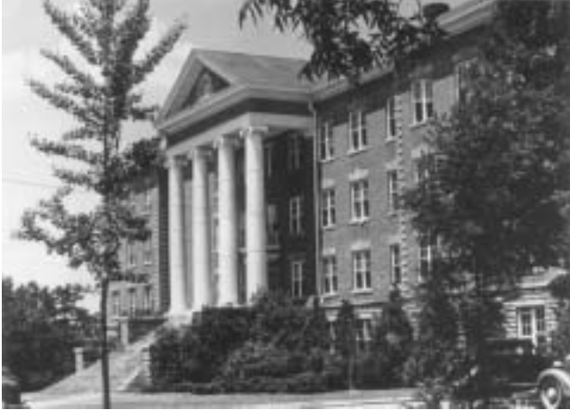
Barracks 3, Front View
