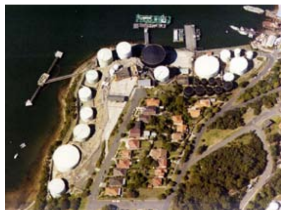
Figure 6. The BP Site in Waverton, in 1991, before demolition. (Photo courtesy NSW Lands Department)
