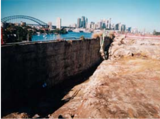
Figure 7. BP Site Waverton, detail of excavation of concrete bund wall. (Photo Courtesy BP Australia)
