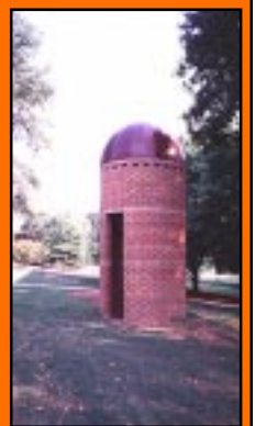
David Tillinghast's silo, located outside Barre Hall
