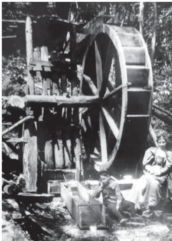
Water-driven stamp mill (ca. 1830-1840), similar to the one constructed under Thomas Green Clemson's supervision at the O'Bar Mine in Dahlonega, Georgia. The Dahlonega Gold Museum.
