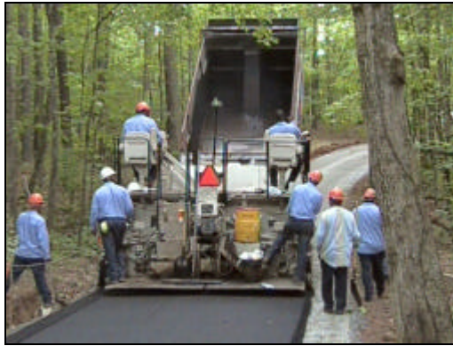
SC Botanical Garden resurfacing provided stunning scenery for the paving crew.
