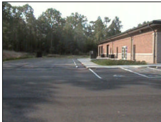
ARTS Research Facility parking lot. Intermediate and surface courses are rubber-modified hot mix asphalt.
