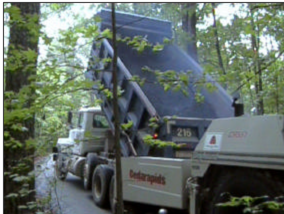
Paving at the SC Botanical Garden.
