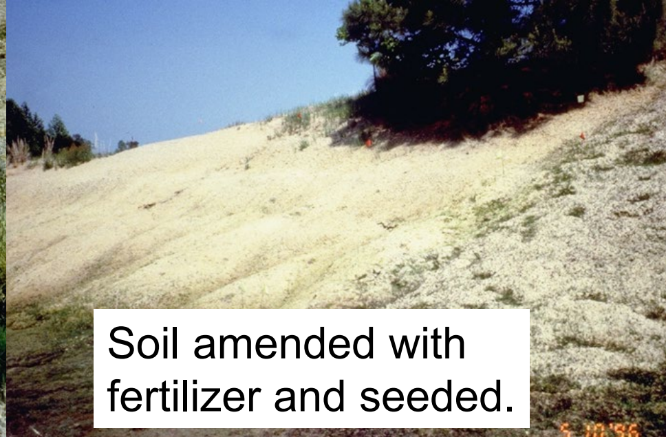
Acid sulfate soil near I-295 in Mechanicsville, VA
