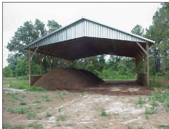
Figure 2. A completed windrow in the composting shed.
