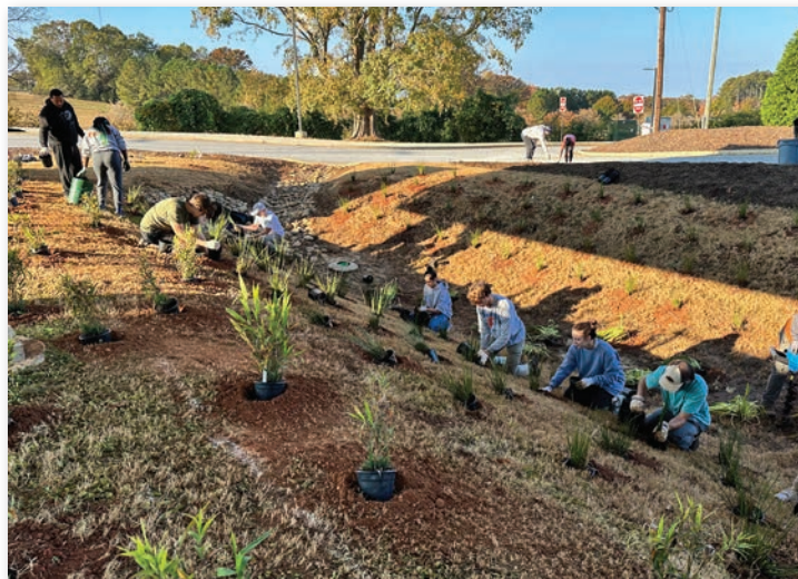
CU students in Landscape Architecture help install plants in a bioretention cell on campus
