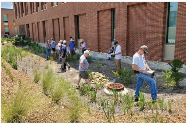
Students inspecting a bioretention cell
