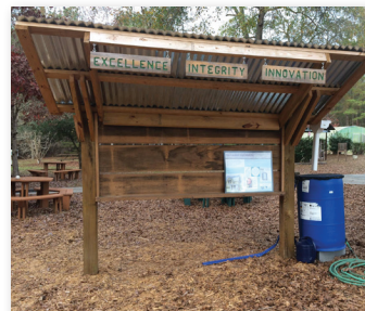
Rainwater harvesting at Central Carolina Technical College.
