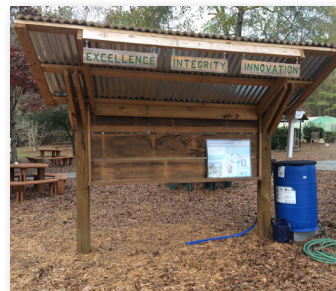
Rainwater harvesting at Central Carolina Technical College.
