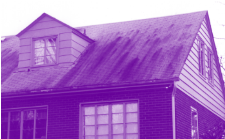
Figure 2. Mildew and algae on shingled roof.
