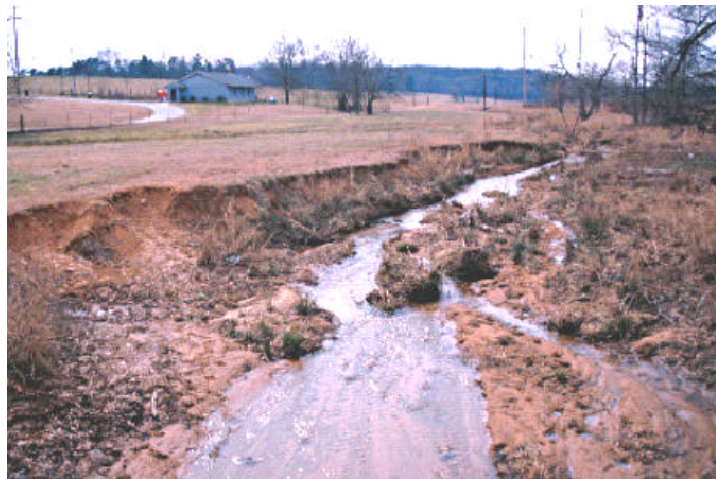
Figure 2-1. Creek in Spartanburg County where open cattle access has resulted in breakdown of banks, channel widening and shallowing with sediment from bank erosion.
