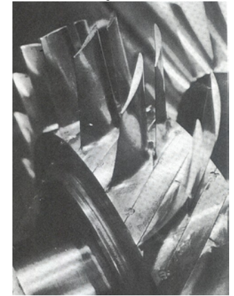
Tandem-Blade Compressor
