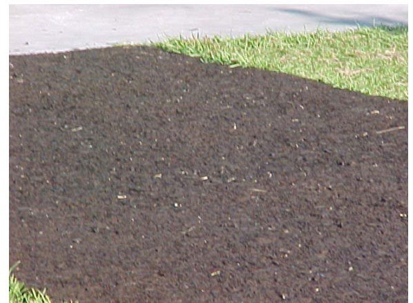
Walkway Made from Waste Tire Chips
