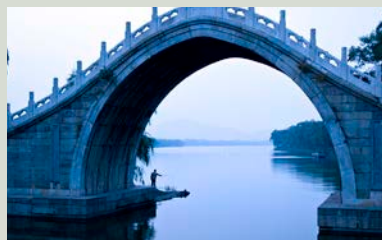
Jade Belt Bridge
