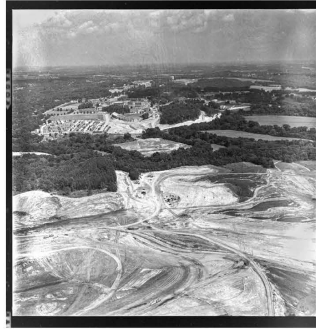
CONSTRUCTION OF DIVERSION DAM NEAR CLEMSON UNIVERSITY
