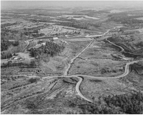
CLEMSON HIGHWAY BRIDGE CONSTRUCTION
