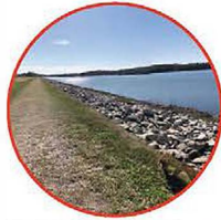
ROWING DOCK LEVEE length - 2,875 ft
