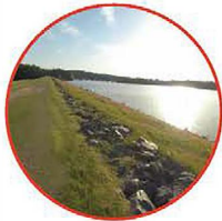
ESO LEVEE length - 2,000 ft
