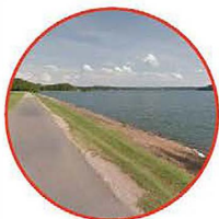
GOLF COURSE LEVEE length - 1,700 ft
