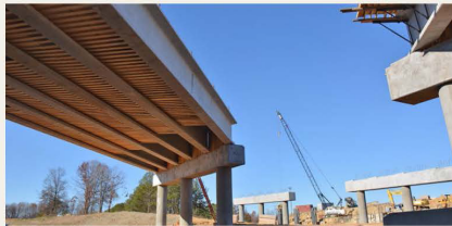
Roads and Bridges
