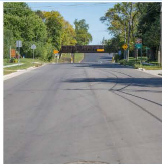
TH 30 Utility Improvements
