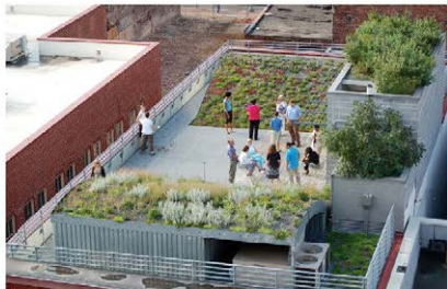
Figure 2 Image of the ASLA green roof with live data results posted on the ASLA website. (Image from ASLA)
