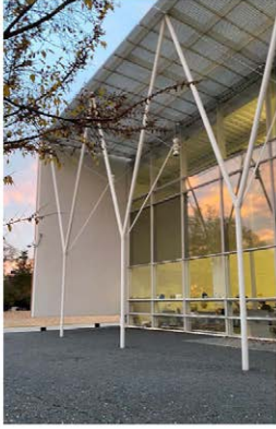
Figure 12b: Exterior columns at Lee Hall.
