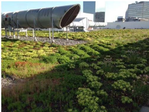
Figure 13 Image of Sam Nunn Atlanta Federal Center green roof ( Greenroofs.com Projects Database - Greenroofs.com )
