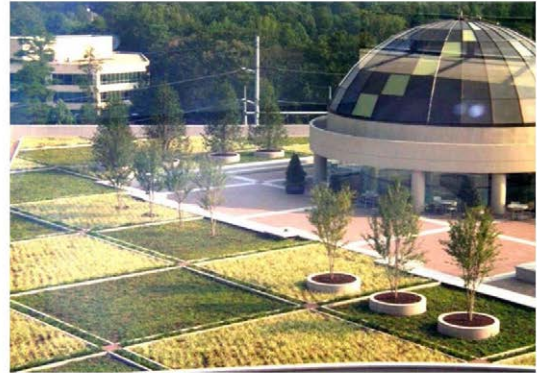
Figure 12 Image of North Park 500 green roof ( Greenroofs.com Projects Database - Greenroofs.com )
