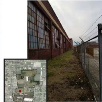
Figure 49: The current state of the building
