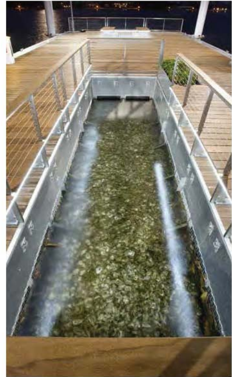
Green ecological sedimentation tank structure. Figure : I. 3.3_1
