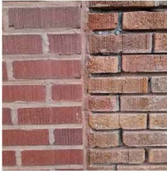
Figure 48: Materiality of the Hoover Complex. Difference of Brick used throughout the building
