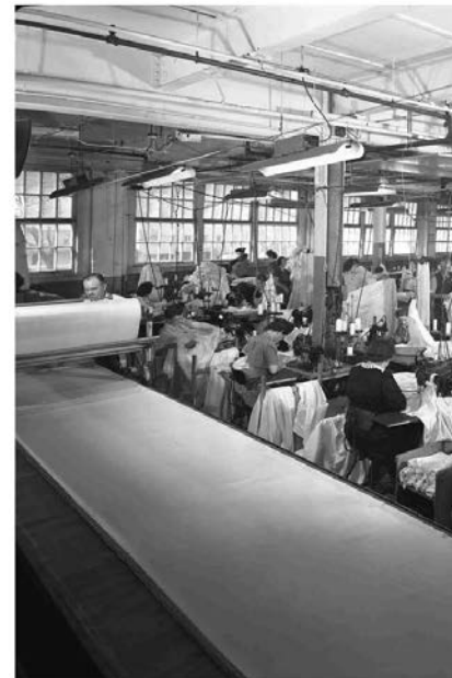
Figure 3: Historic photo inside the Hoover Company Factory
