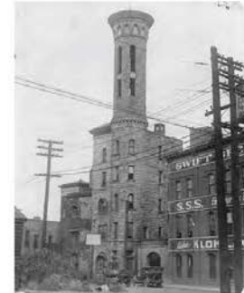
Figure : III.1.1_6 Fulton County Jail abandoned by the city in 1960 when a new jail was opened on Jefferson St. Demolished in 1962.
