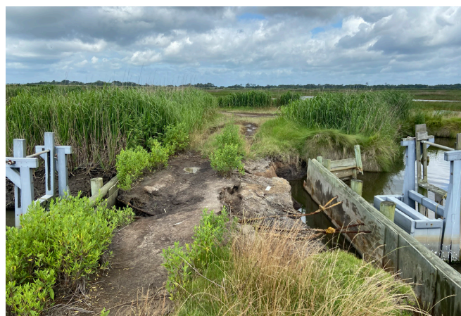
Figure 2: Damaged earthen dike and wooden trunk due to sea level rise and tropical storm events.
