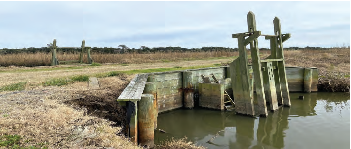
Figure1: Historic wooden trunk (flapgate structure) used for water level management in managed antebellum rice fields along the South Carolina coast. These traditional structures continue to play a vital role in wetland management, supporting waterfowl habitat and maintaining ecological balance.
