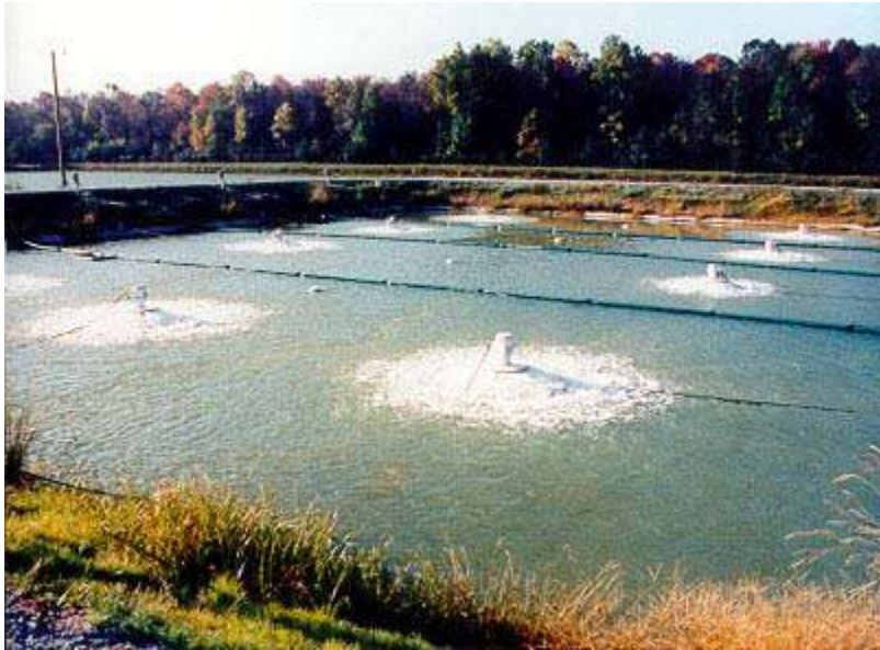
Figure 3. Photograph of a DPMC aerated lagoon system
