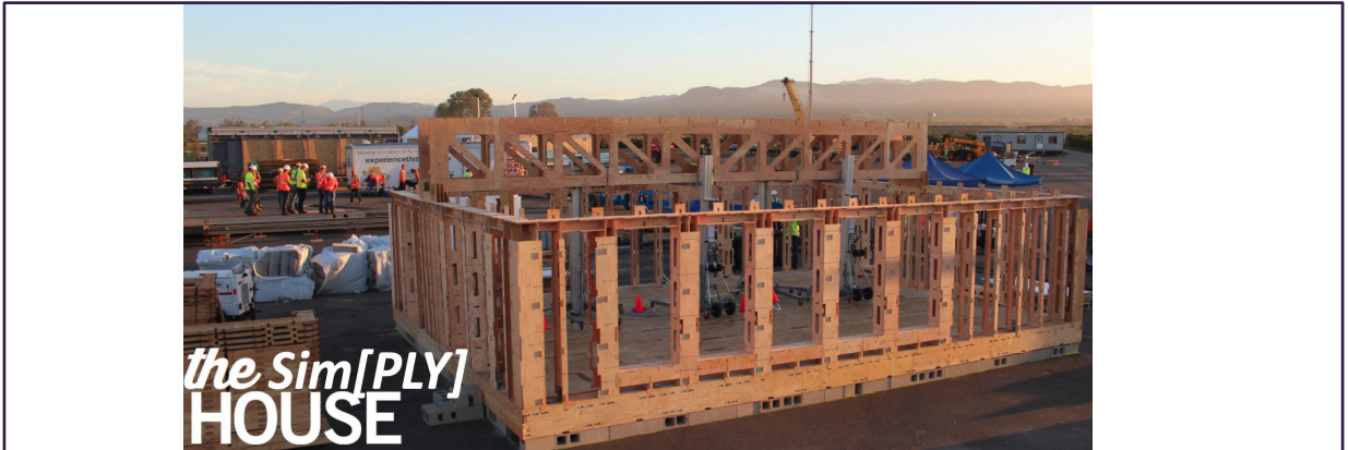
Patented Building Construction System: Sim[PLY] CNC-cut plywood assembled as 3D puzzle held in place with metal zip ties
