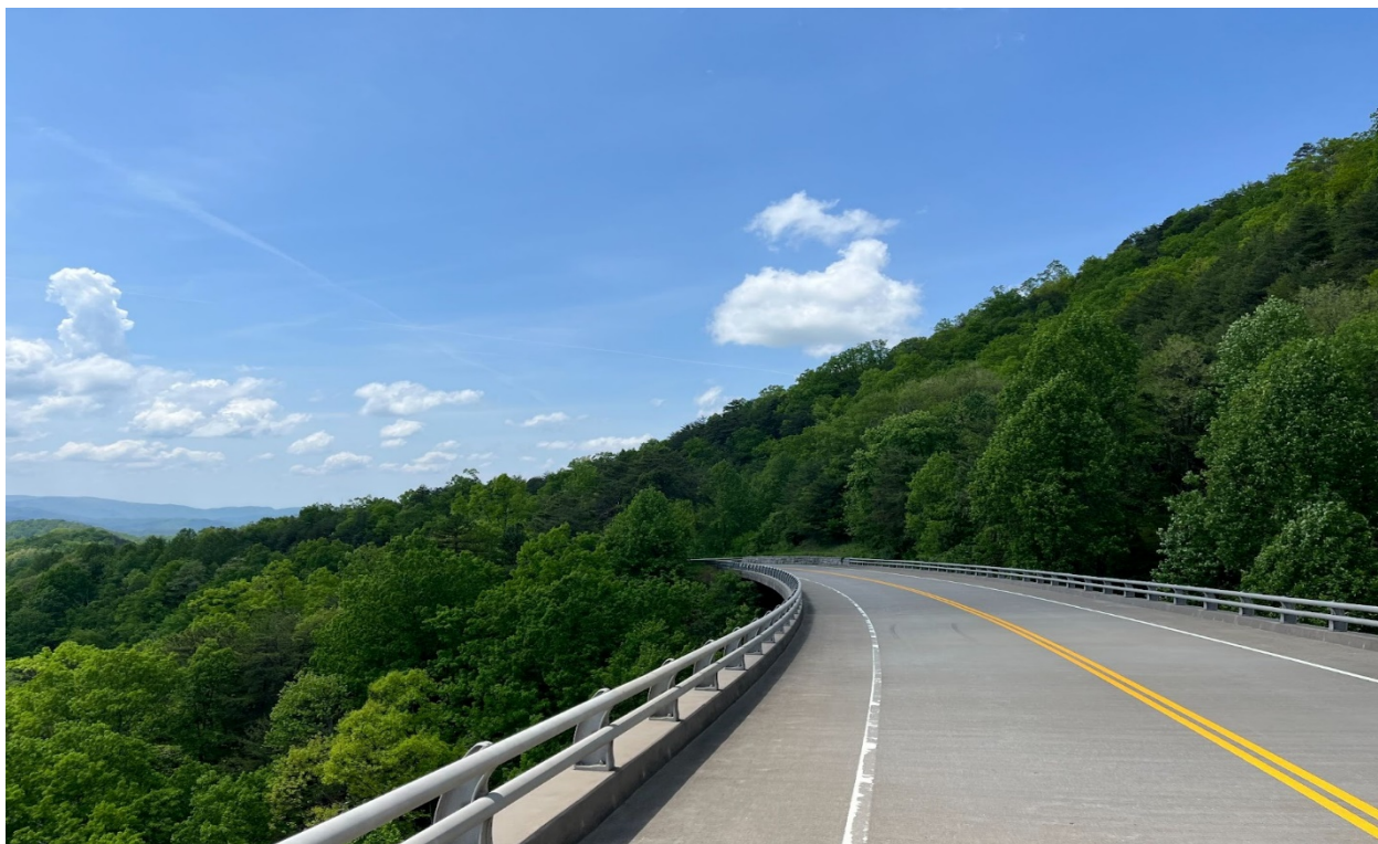
Foothills Parkway viaduct near Rocky Mountain
