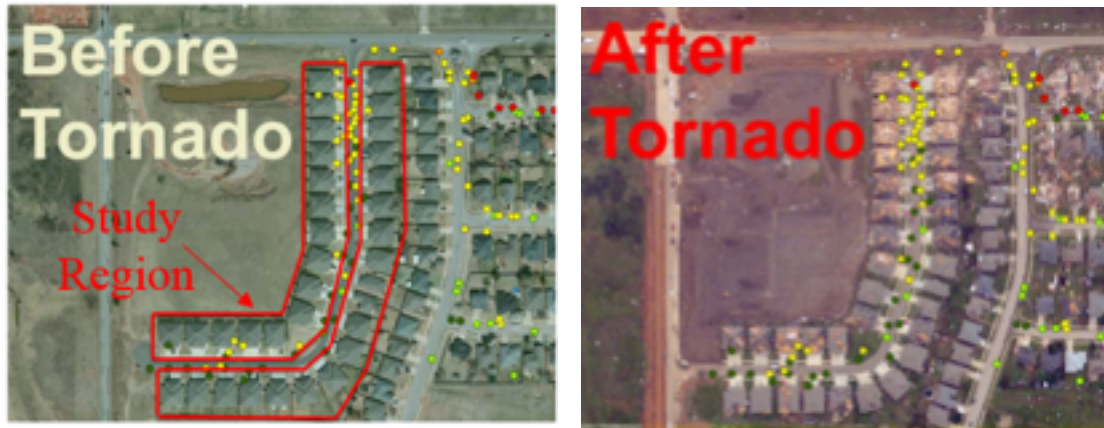
Figure 1: Tornado induced damage for residential light-frame wood structures (Adapted from Dao et al. 2014)
