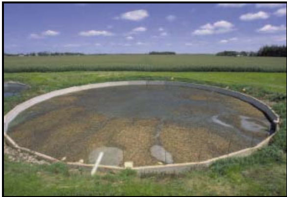
Figure 2. A biocover formed by a layer of chopped corn stalks on the surface of swine manure (Lorimar et al., 1998).
