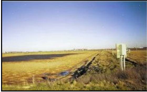
Figure 6. Combination cover made of geotextile and a layer of straw (Lorimor, 1999a).
