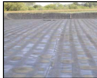
Figure 5. A two-layer geotextile cover with additional floatation provided by a layer of closed cell foam (Nicolai et al., 2004).
