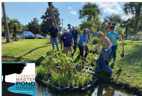
Floating Wetland Installation
