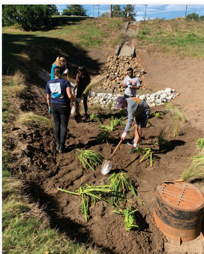
CU students and staff installing a bioretention cell as part of Solid Green Day.
