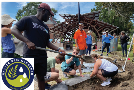
Rain Garden Installation
