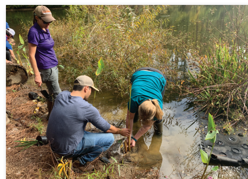
Installation of Shorescape
