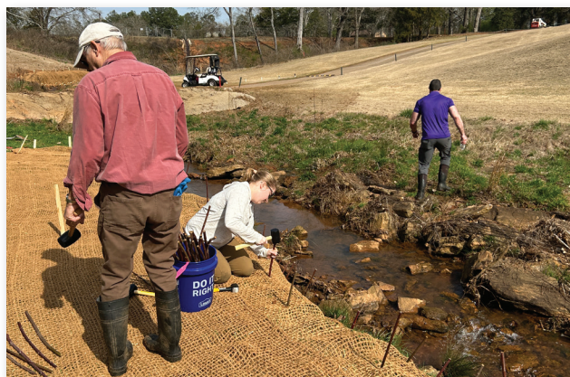
Workshop participants installing native livestakes to revegetate stream bank
