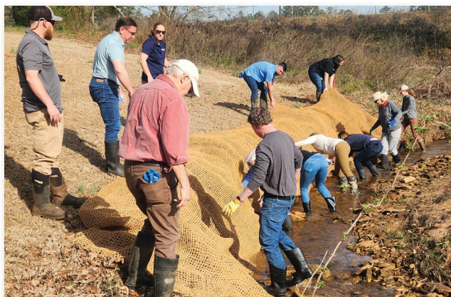
Workshop participants anchoring erosion control matting to stream bank
