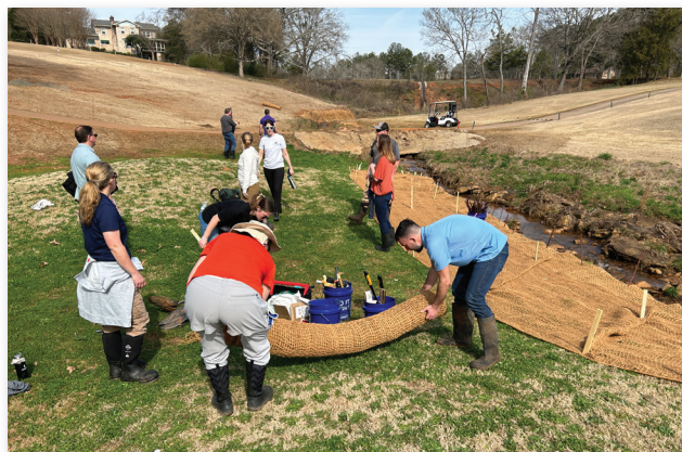
Workshop participants rolling out erosion control matting
