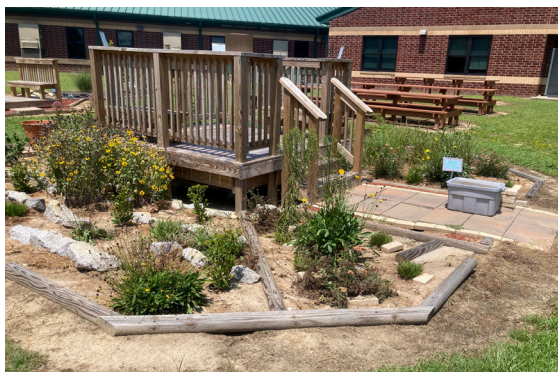
Native plants are used for water filtration in bioretention cell installation at Darlington Middle School's Environmental Awareness Center.
