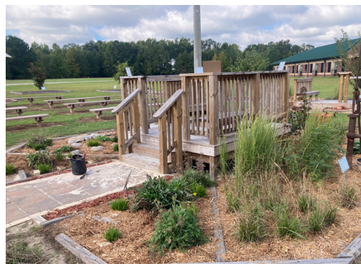
Native plants are used for water filtration in bioretention cell installation at Darlington Middle School's Environmental Awareness Center.
