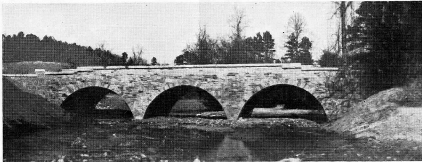
Spanning Six Mile Creek, this triple-arched bridge on the Park Road was constructed entirely by relief labor, and largely with native materials
