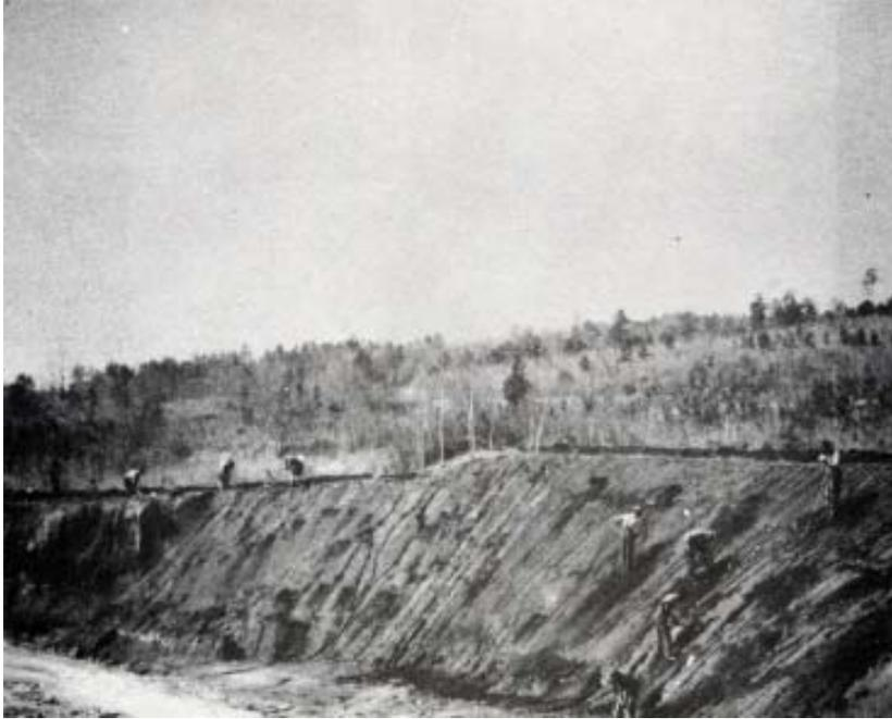
*Figure 16. WPA workers planting kudzu for erosion control.*
