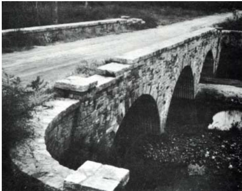
*Figure 10. Triple-arched stone bridge spanning Six Mile Creek. Built by WPA, 1939.*
