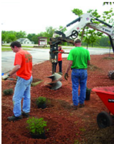
Digging a hole for a shrub with a bobcat
