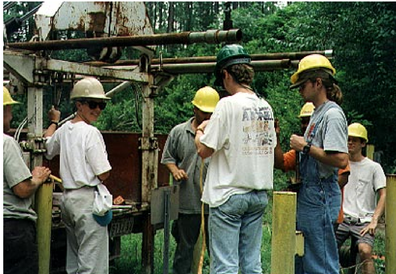
Setting a well pump during the Clemson Hydrogeology Field Camp
