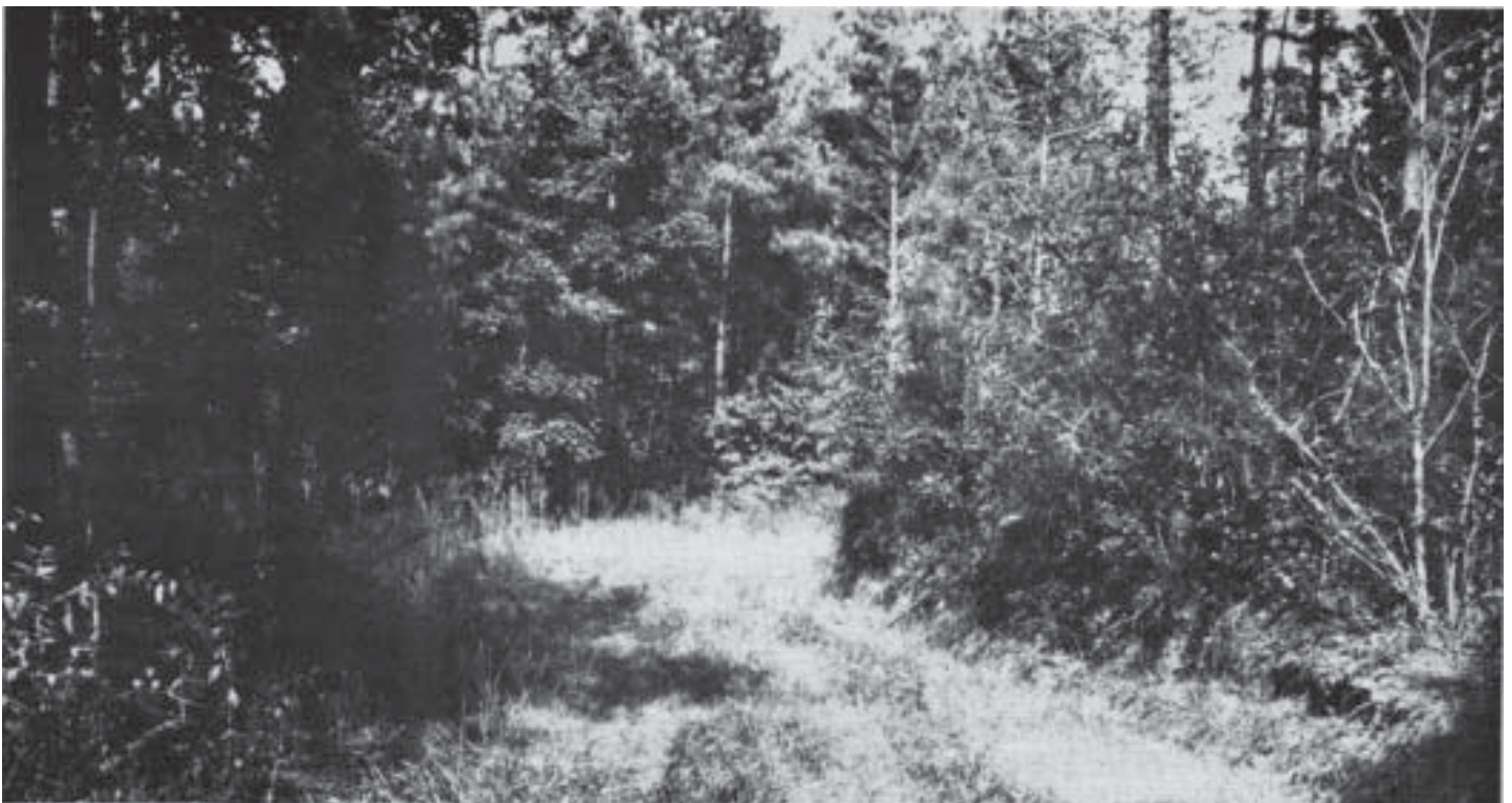
An example of road stabilization. This road “paved” in grass helps prevent runoff from rain.
