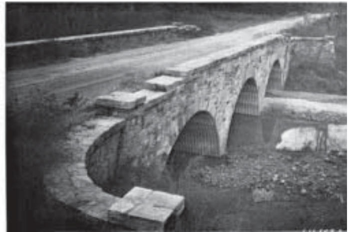
This triple-arched bridge over Six Mile Creek was built of native materials by relief labor.
