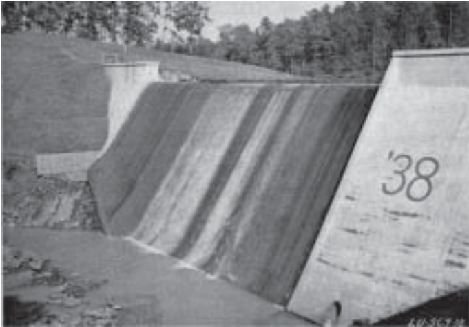
The concrete dam and spillway at Lake Issaqueena.
